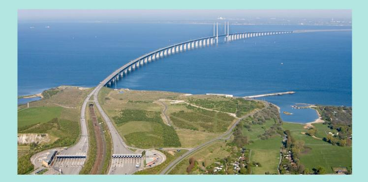
What is colloquially known as the Öresund Bridge consists of a bridge, an artificial island and a tunnel, and the entire link is 16 kilometres long. The combined road and rail link was completed in 2000. Some seven million vehicles use the link each year, of which approximately 90 per cent are passenger cars.
